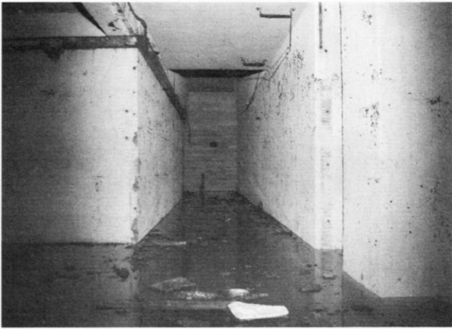
The entrance dogleg and transformer bay. Photo by Gavin Saxby
